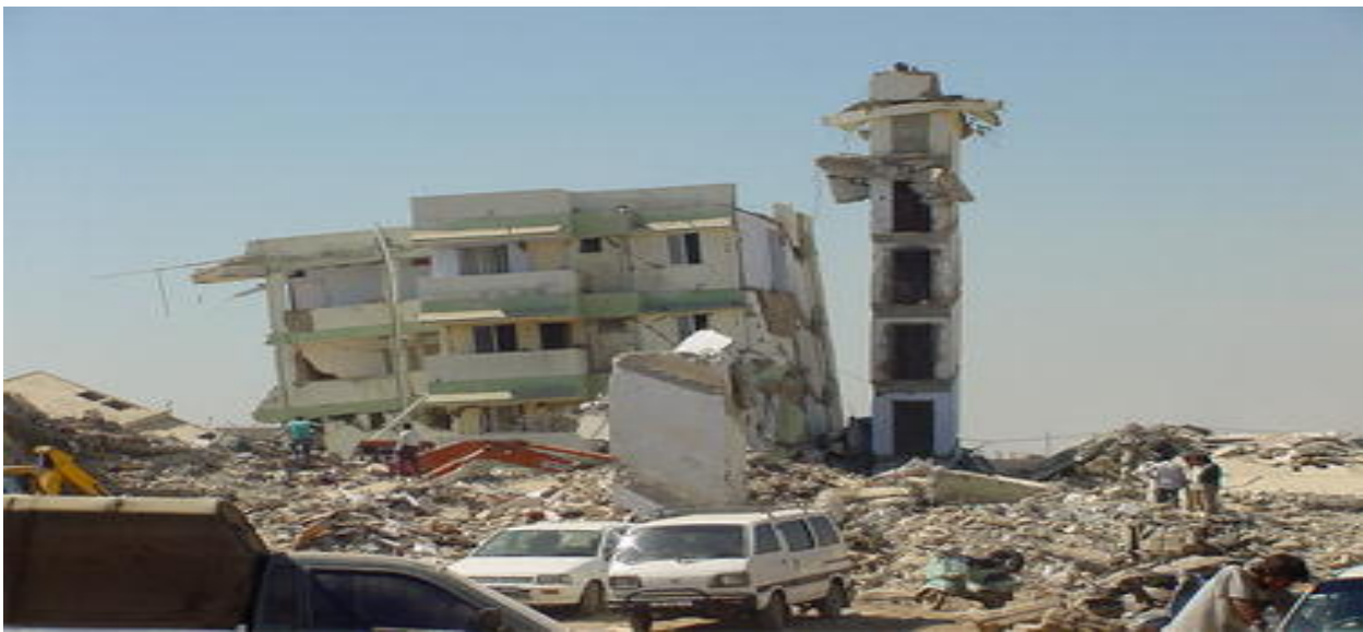
Figure 1: Apartment collapse in bhuj (2001).
