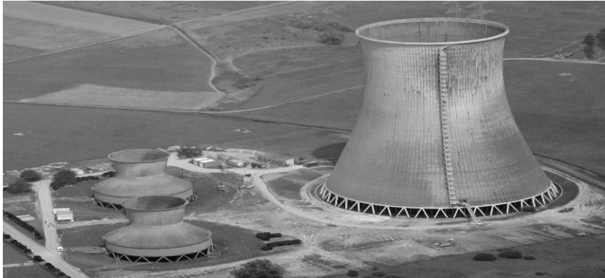
Figure 4: Industrial cooling tower at a power station.
