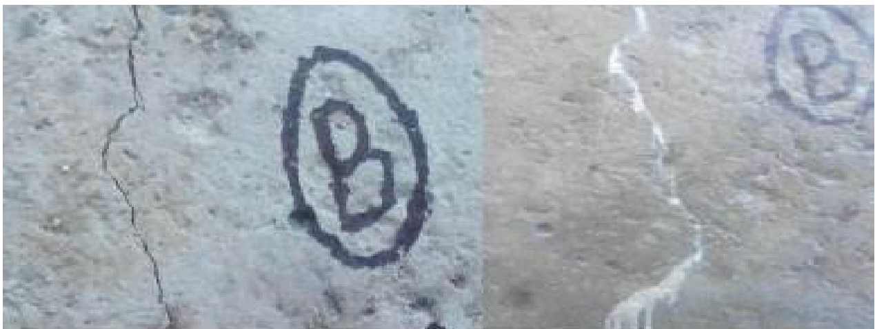
Figure 6: Self-healing of cracks developed.
